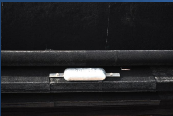
Zinc anodes are applied on top of foil
